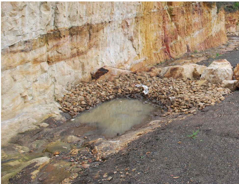
Figure 6-1 Typical in-line rock check dam
