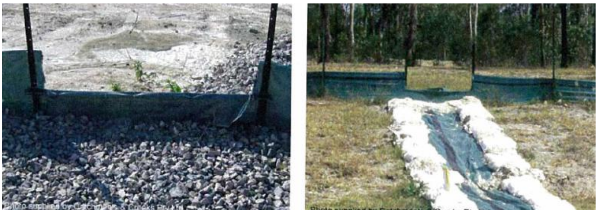
Figure 1 Spill-through weir outlet options (catchments and creeks)
