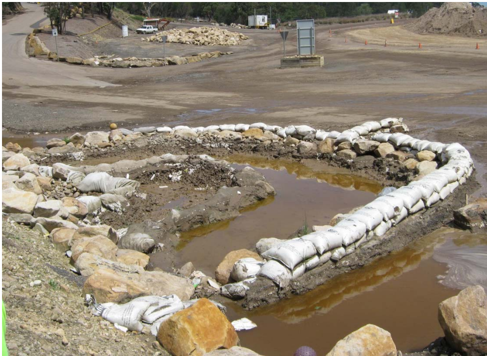
Figure 6-2 Typical drain entrance rock check dam from large disturbed area
